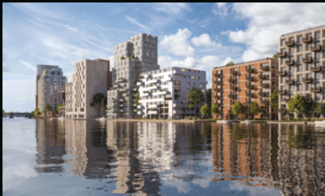
Flour Mill Mixed Use Re-development (Amsterdam, NL)
